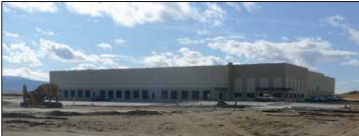
Construction of American Tire Distributors
